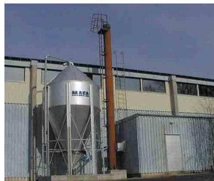
Inside and outside pellet storage installations.
